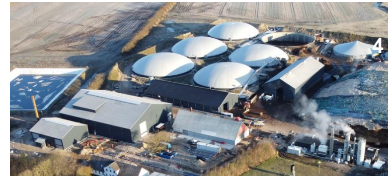
Q1 2024: 20 MW plant starts operating at BB Energi.
