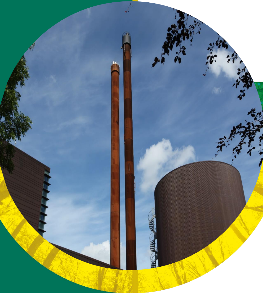
Skive District Heating Plant, Denmark Photo: Torben Skøtt
